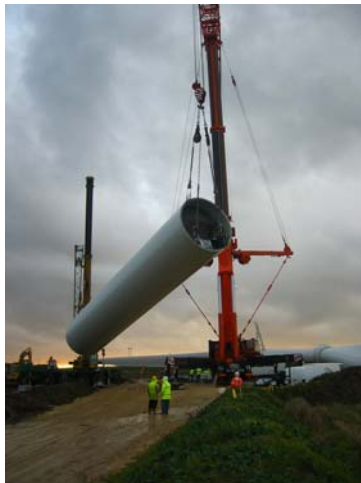
The bottom tower section being raised into the vertical position prior to being placed on the embedment cylinder. The rotor assembly can be seen in the background.
