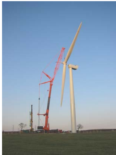
The two tower sections and nacelle are in place and the rotor assembly is lifted into position.
