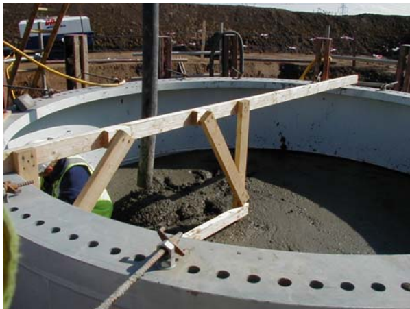
Concrete being levelled inside the embedment cylinder. Note the lower tower section is bolted to the embedment cylinder via the holes seen in the foreground.
