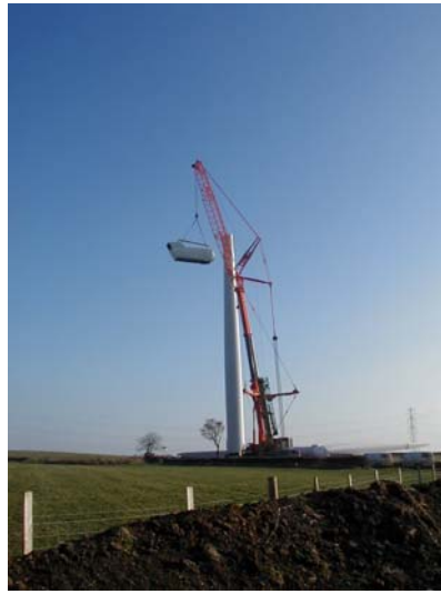
The nacelle is lifted into position at High Volts.
