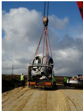
This shows the centre hub of the rotor assembly being delivered. The 3 blades are bolted to this hub on the ground and the complete rotor unit is lifted by crane and attached to the nacelle.
