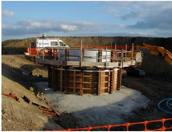
This shows the circular plinth shuttering in position prior to the plinth being poured at Holmside. Note the steel embedment cylinder protruding from the top.
