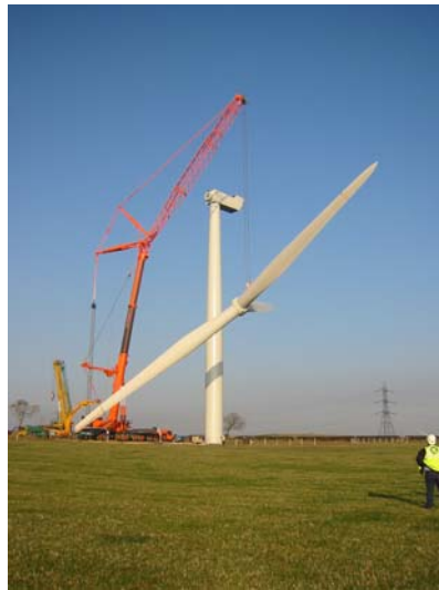
The two tower sections and nacelle are in place and the rotor assembly is lifted into position.
